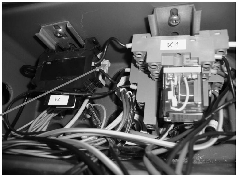
Protective grounding conductor, mounted underneath the two fuses F2 and F3.
